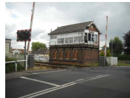
Plate 11 View towards the signal box
