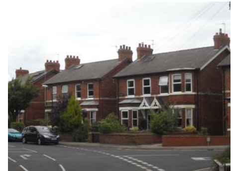
Plate 4 View of houses on the north side of The Village
