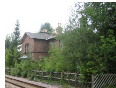
Plate 12 The former station house
